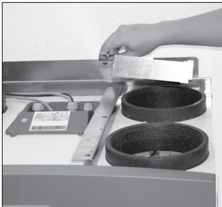
4. Attach the mountings to the U-profile
