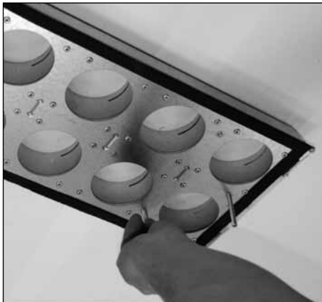
1. Screw in threaded rods
