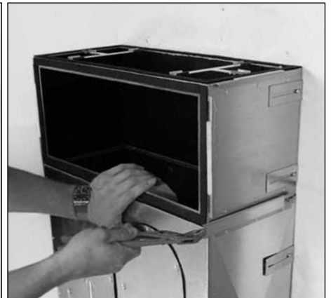
3. Pull off clamping rail
