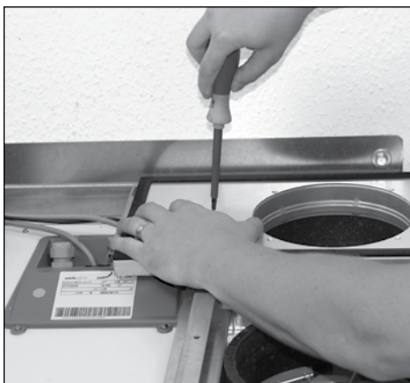
7. Secure end piece plate with one screw
