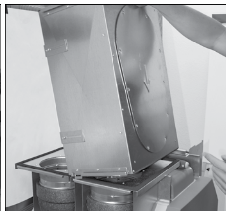
9. Place ComfoWell on the end plate
