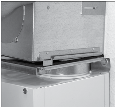
4. Mount ComfoWell on the end plate
