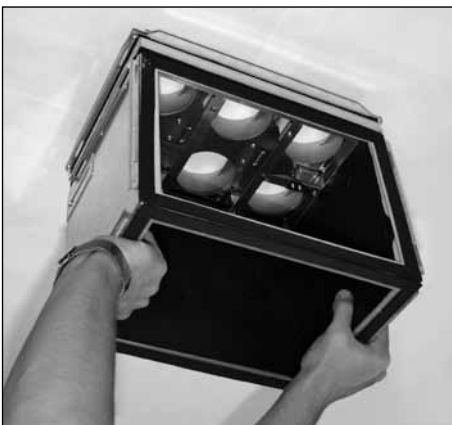
4. Push manifold onto the threaded rods until the manifold locks in place
