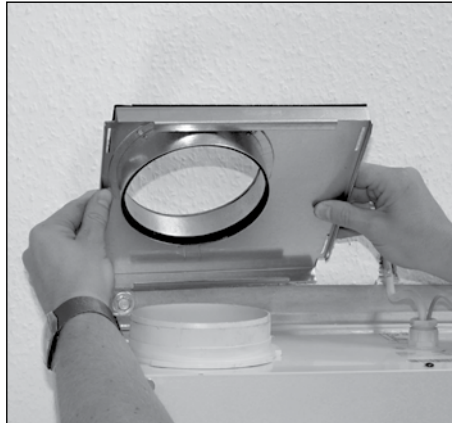
2. Attach end plate to CA 140
