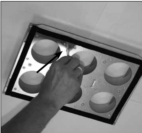
1. Screw the threaded rods into the mounting plate
