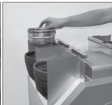
6. Insert the 160 mm nipple into the CA 350
