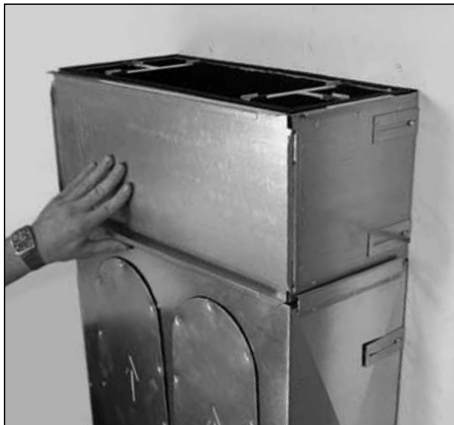
1. Pull off clamping rails
