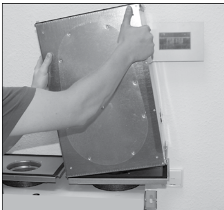
4. Place attenuator on the end plate
