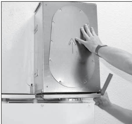
4. Mount ComfoWell on the end plate
