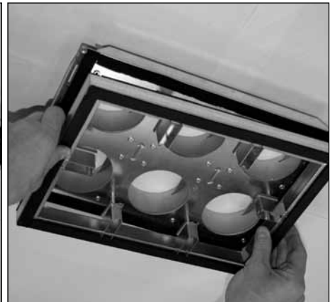
3. Push the spacer frame onto the threaded rods
